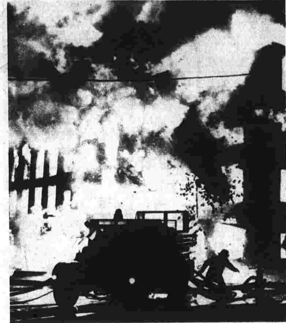
Fire Collapses Wall
